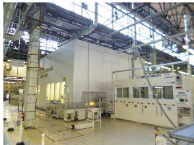
Fig. 7 Overall view of MS peening process
