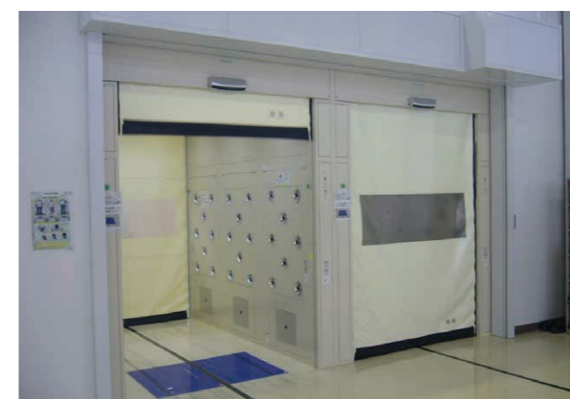
Fig. 2 Installation of double shutters and air shower at parts entrance
