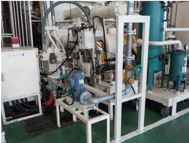
Cold water circulation equipment at forging facilities
