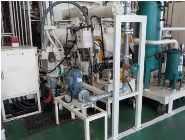
Cold water circulation equipment at forging facilities
