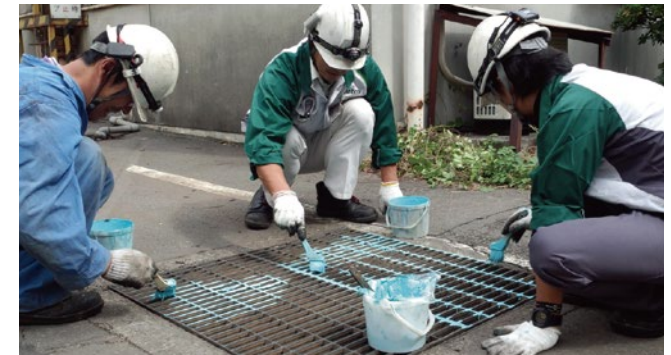
Color-coding of drainage outlets by employees
