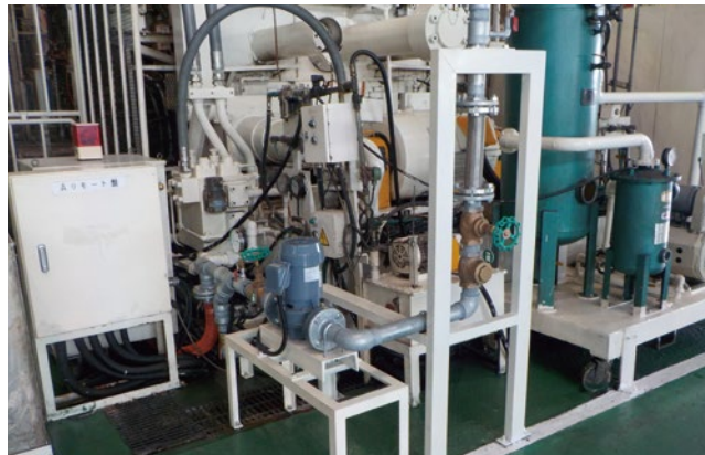
Cold water circulation equipment at forging facilities
