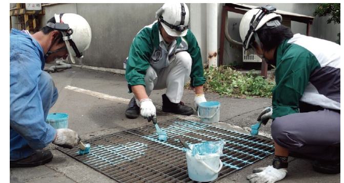
Color-coding of drainage outlets by employees
