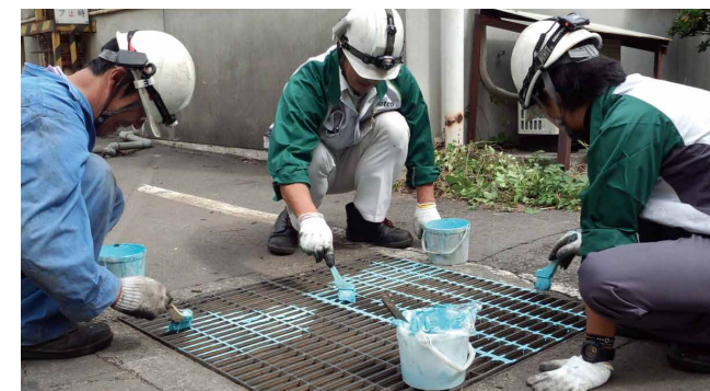
Color-coding of drainage outlets by employees
