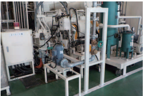
Cold water circulation equipment for forging facilities
