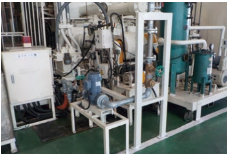
Cold water circulation equipment for forging facilities
