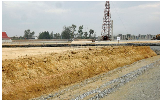
Building site where the filling was carried out
