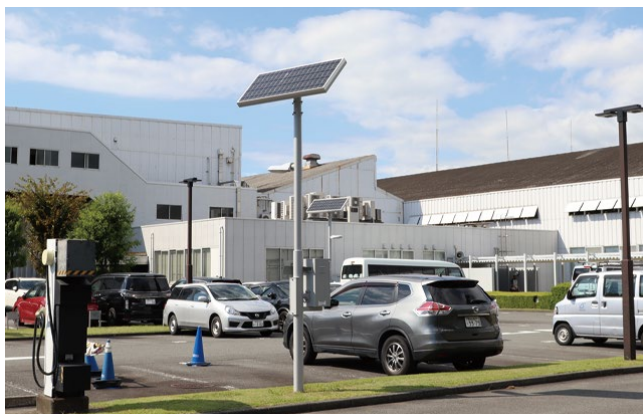
Solar powered outdoor lighting being installed at Fuji HQ
