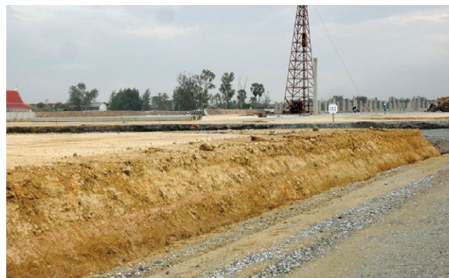
Building site where the filling was carried out
