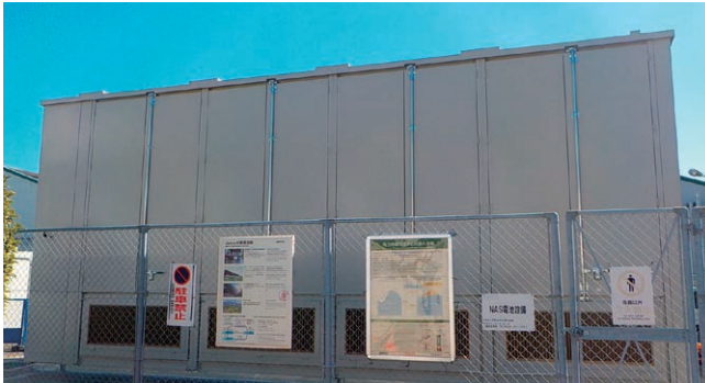
NaS battery facility *NaS battery: A storage battery composed of liquid sodium (Na), liquid sulfur (S), and special ceramics
