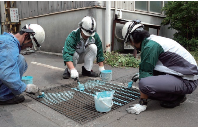
Color-coding of drainage outlets by employees
