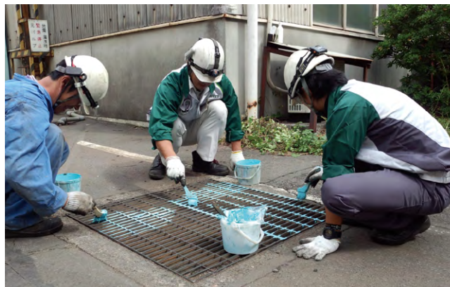
Color-coding of drainage outlets by employees
