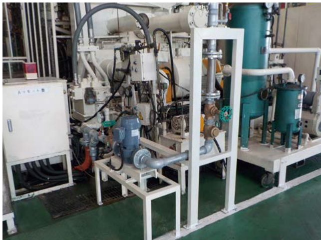
Cold water circulation equipment at forging facilities
